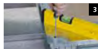
3 Level with the screws
