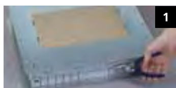
1 Cut the trunking entries
