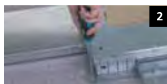
2 Insert the trunking and screw to floor
